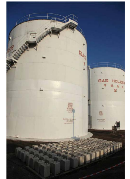
Energy recovery from sewage treatment plant & steel mills
